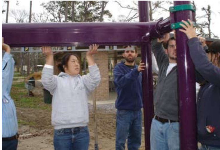
Assembling Playground Equipment: CEE students Lauren Huey (2nd from left) and Brandon Kluzniak (3rd from left)
