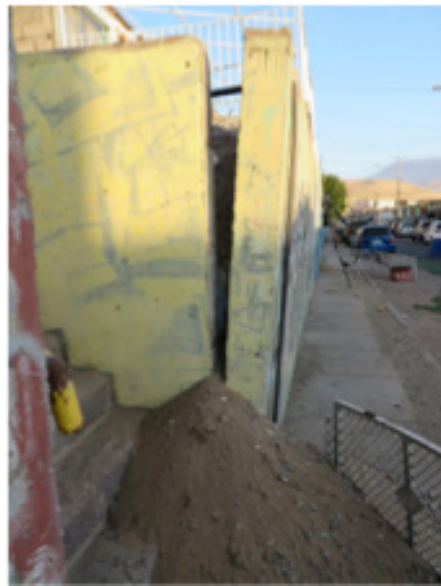
Figure 3. Reinforced concrete wall without a footing rotated during the 2014 Iquique, Chile, earthquake. Courtesy of G. Candia
