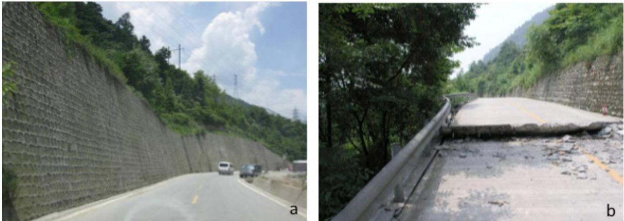
Figure 2. Conventional retaining structures in the epicentral region of the Wenchuan 2008 Earthquake. Note the fault break in the picture on the right.
