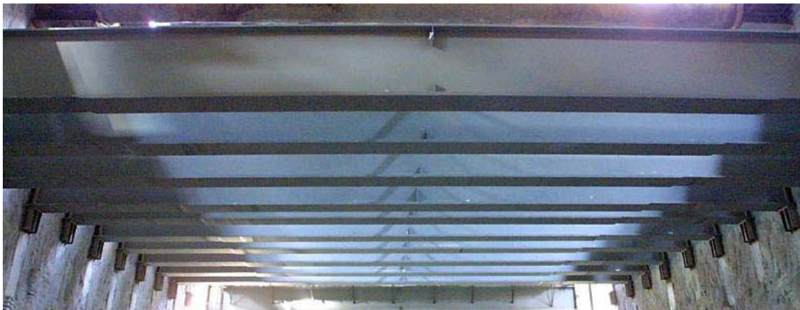
Figure 2: Photo of as-built soldier-pile tremie-concrete slurry wall and composite steel-and-concrete roof system
