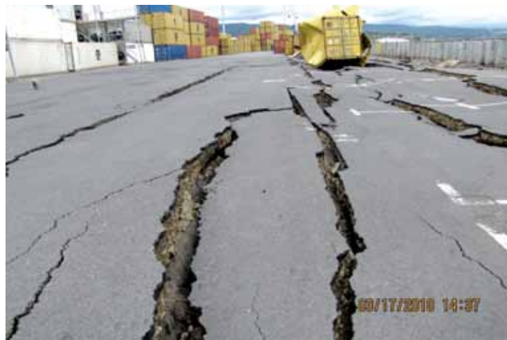
Liquefaction and Lateral-Spreading Induced Damage at the Port of Coronel (GEER, 2010; S37.0287°, W73.1500°; 03/17/2010)
