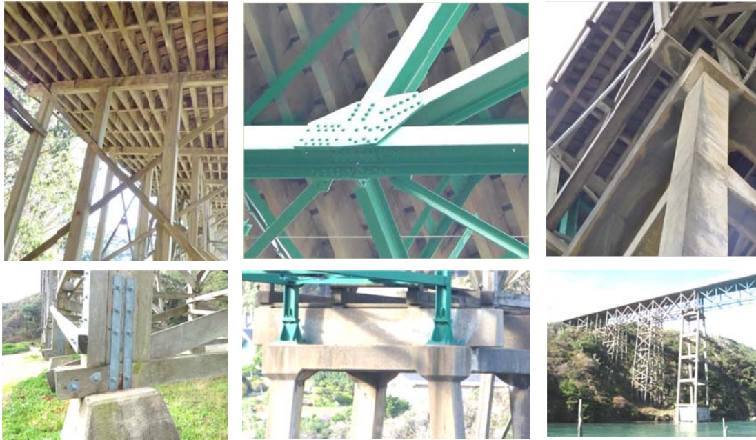
Figure 11: Close-up Views of Typical Timber, Steel and R/C Parts of the Albion River Bridge
