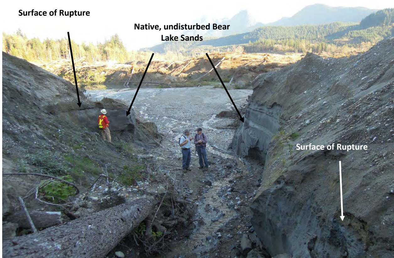
1 2 Figure 9: View of surface of rupture exposure with clay shear zone at top of Bear Lake Sands (photo taken on 3 10/23/2015 at 48.282N;121.848W, looking SW). 4
