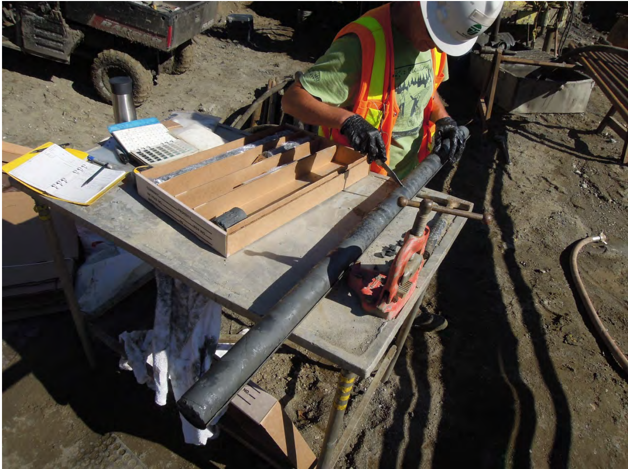
1 2 Figure 7: WSDOT Inspector examining soil core sample and packaging in core box. 3
