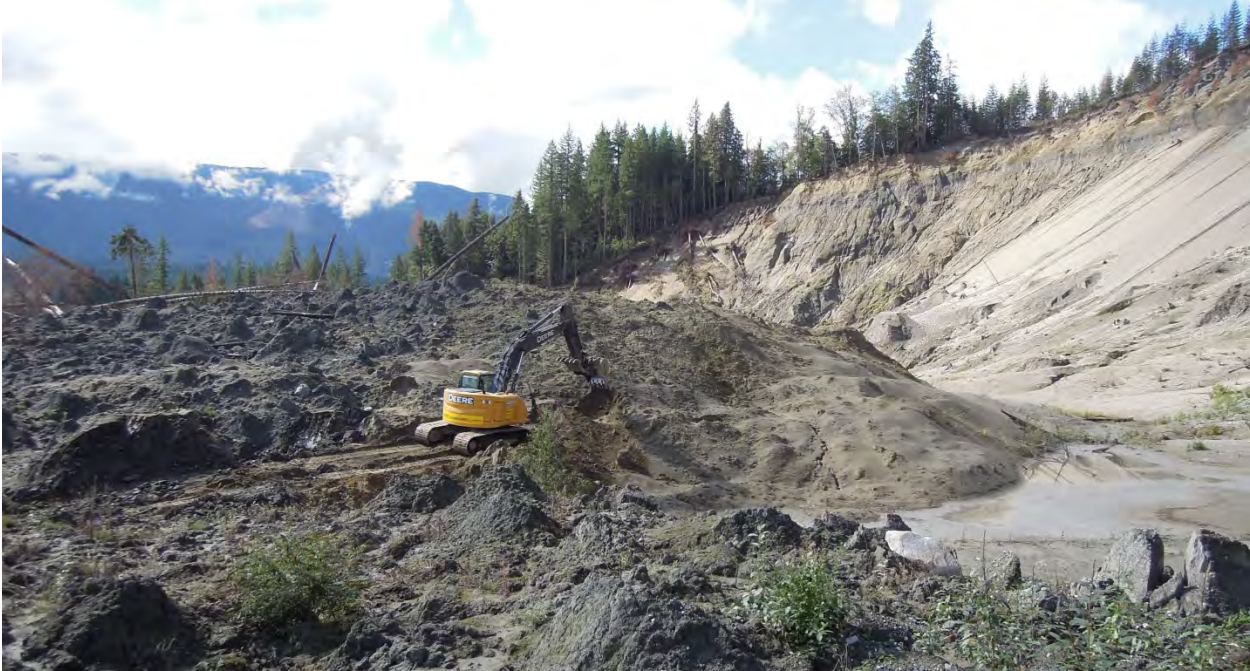
1 2 Figure 5: Tracked excavator grading an access path to the drill pad for EB-04 on the main body of SR 530 Landslide. 3
