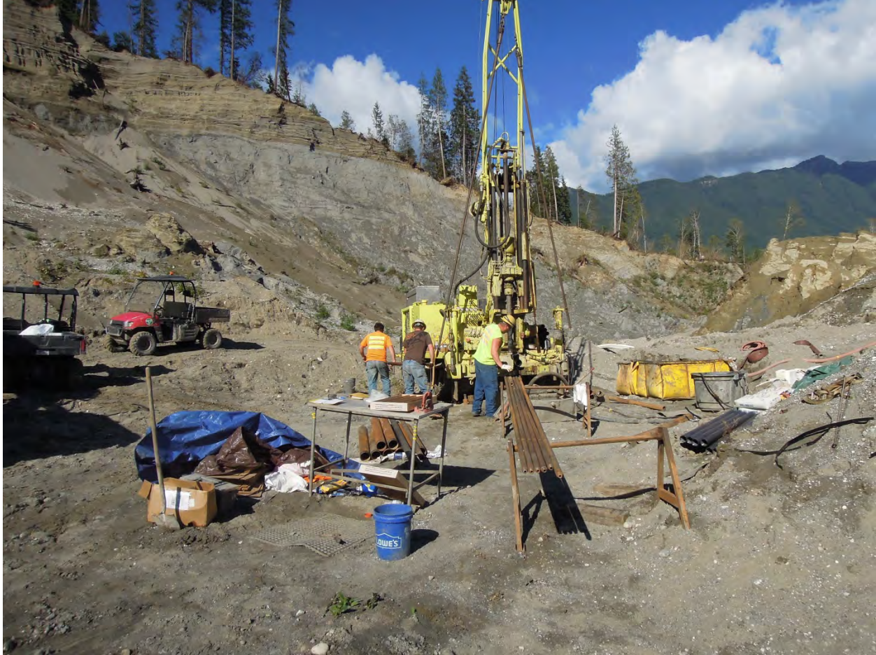
1 2 Figure 6: CME-850 drill rig setup at EB-04 on the main body of SR 530 Landslide (drill rods supported on stands). 3
