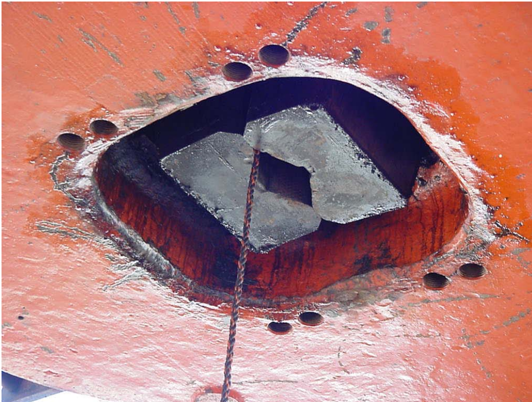
Turn on the grips. Using the crane and a cable insert spud through grips.
